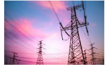
AI Consumes Considerable Electricity and Chilled Water
